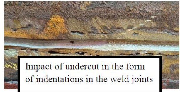
Figure 4: Undercut welding defect
