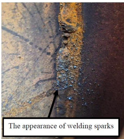
Figure 6: Spatter welding defect
